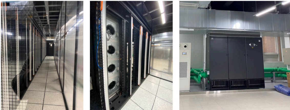
Fig. 3. Images of the containment system, CRAH, and water-cooled chiller in the reference containment data center.
