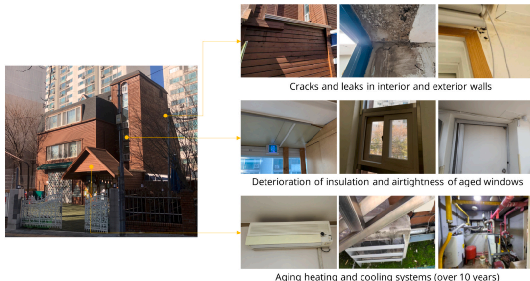
Fig. 4. Photos of the field survey of the target building.
