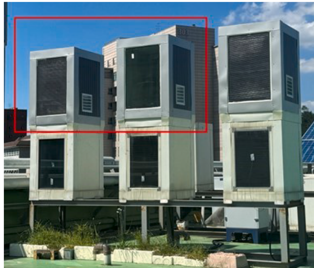
(a) Photograph of the mock-up installation.
